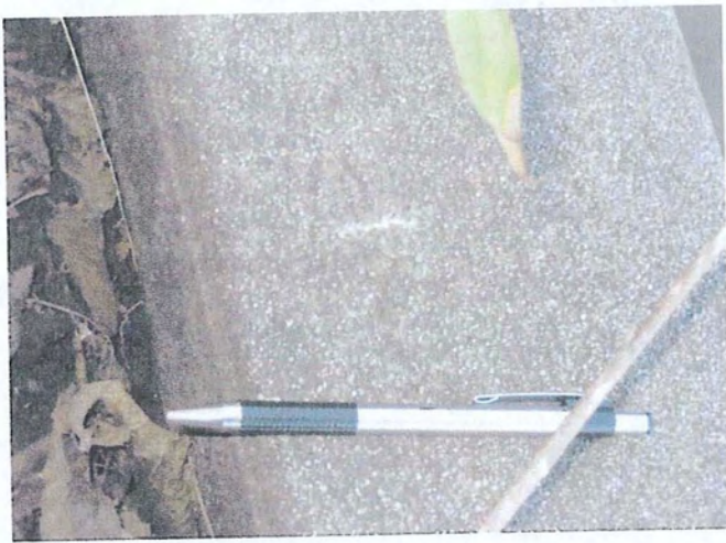
Scratch mark located on outside portion of top of wall. Pen shows its relation to mark in above photo
