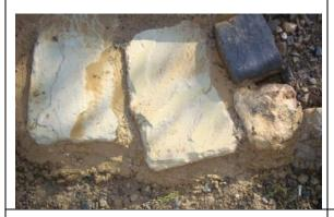
20. The Concrete mixed with cement color was poured inside the boulder 'structure" and directly on the ground around the rest of the tub. The stepping stones were set in the colored concrete around the tub, creating a ledge.
