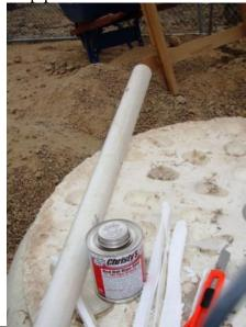
8. In construction, white pipe is used for the incoming clean water, and the black pipe is used for the outgoing dirty water. Since we only use bleach to clean, we used mostly white pipe.
