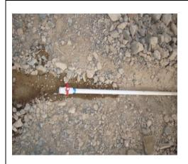
11. Once the pipe is tested for leakage, it is then buried under the soil. The only thing left exposed is the valve to drain the tub.
