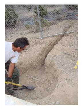
4. The hole is dug in the shape of the tub. The ditch for the drain pipe continued to the outside of the cage, so the animals can't get to it and chew on the drain valve.
