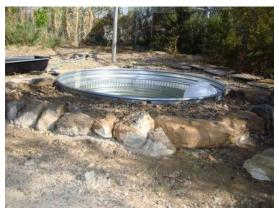
19. Next we sprayed our rock structure with water to prepare it for the pouring of concrete.
